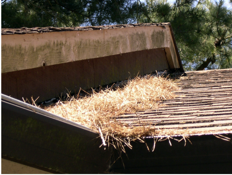
Figure 5. Vegetative debris accumulated at this roof-to-wall intersection. Ignition of this debris would expose the adjacent siding to flames, as well as the underlying sheathing above this stand-alone Class A roof covering. Depending on the overall roof design, the Class A roof covering could give the homeowner a false sense of security. Photo: Stephen L. Quarles.
